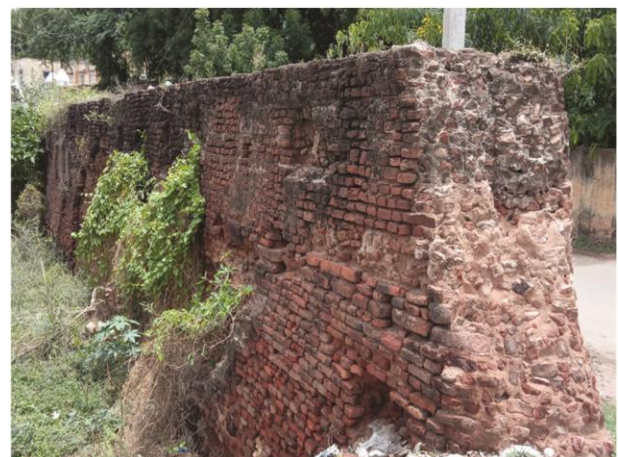
Fig. 7 — A 1.2 m wide rampart wall with brick courses in the upper portion
