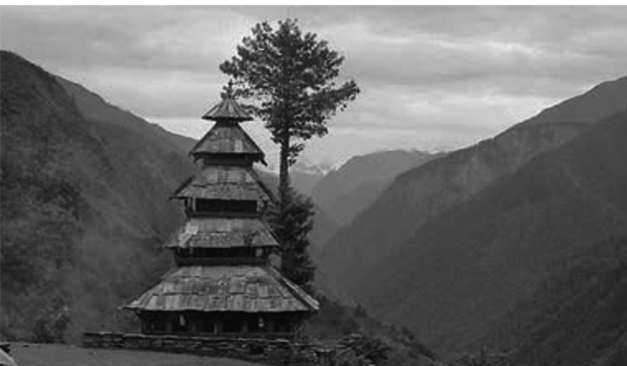
Fig. 6 — Manu Temple at old Manali showcasing multi-tiered Pagoda style roofing and Kath-khuni style construction (Beas valley) (Source: by Christina Noble at British Museum)
