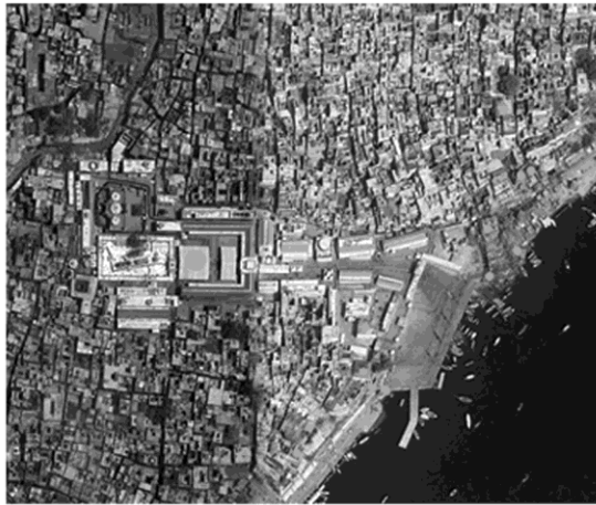
Plan of Varanasi, showing a cluster of centrally located temples. The temples are grouped together in one region, surrounded by the bustling town streets.
