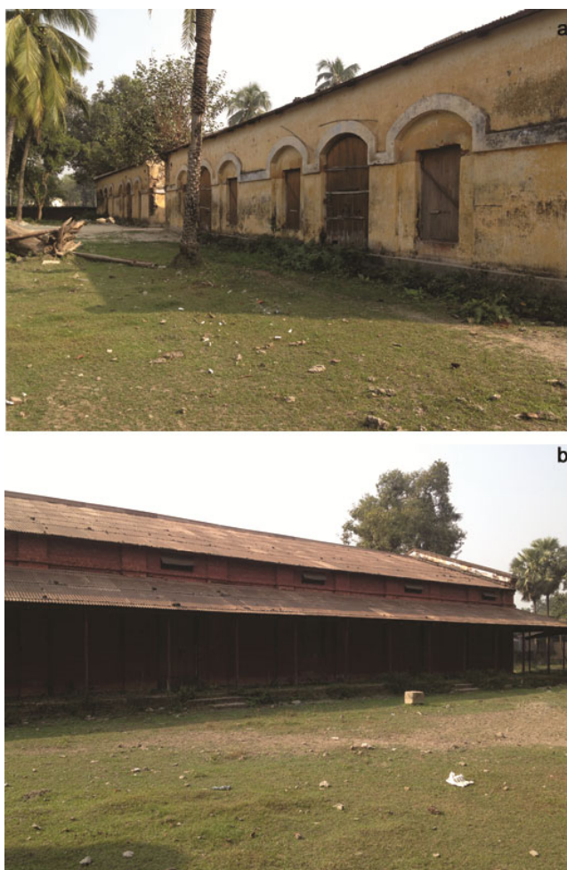
Fig. 4 — Photo: a) Ganja society's storage facilities at Muktir More, Naogaon, and b) Ganja society's storage facilities at Muktir More, Naogaon.
