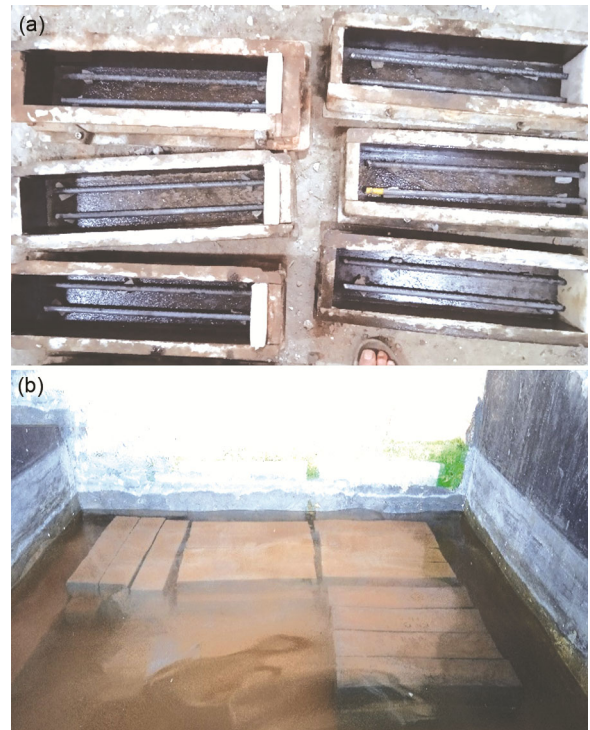
Fig. 4 — (a) formwork for RCC beam. (b) beam samples in the curing tank.
