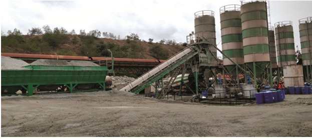
Fig.4 — Arrangement of hoppers and silos in the batching plant.
