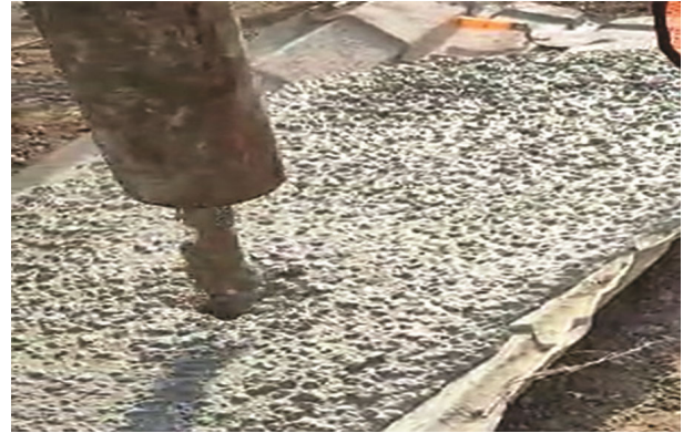
Fig. 13 — Cohesive AAC mix at pouring location.
