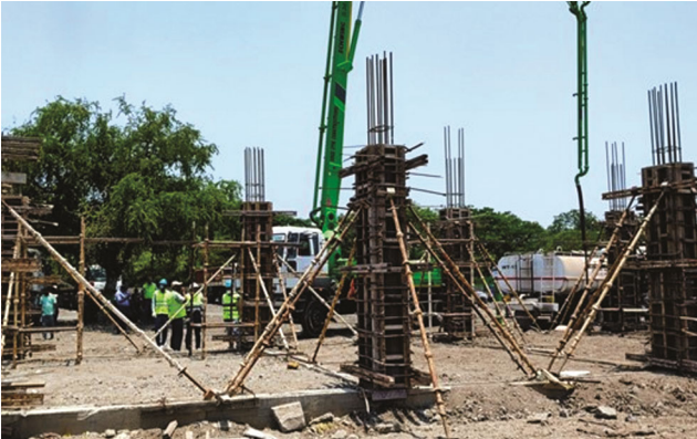
Fig. 8 — Pouring of concreting using a truck mounted boom placer pump.
