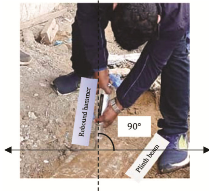
Fig. 10 — Rebound hammer testing of the plinth beams of substation.
