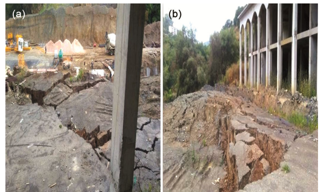
Fig. 6 — Morphology of landslide (a) Visible cracks in the ground and (b) Ground collapse.
