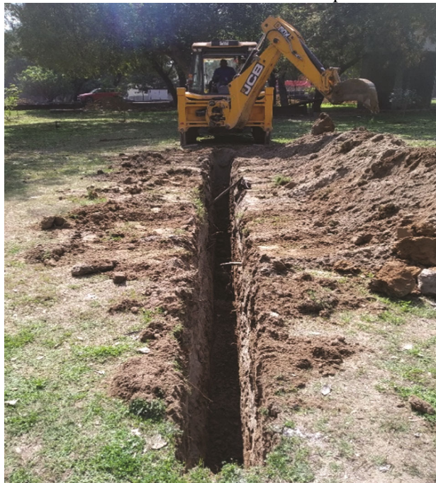
Fig. 2 — Formation of trench at test site location with JCB excavator.
