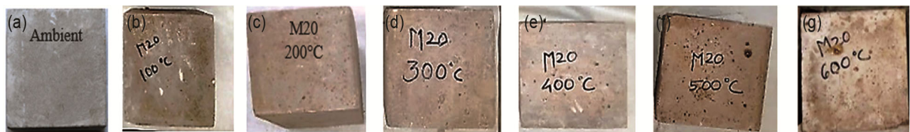
Fig. 3 — Concrete cubes after thermal exposure to elevated temperatures. (a) Ambient, (b) 100° C, (c) 200° C, (d) 300° C, (e) 400° C, (f) 500° C and (g) 600° C.
